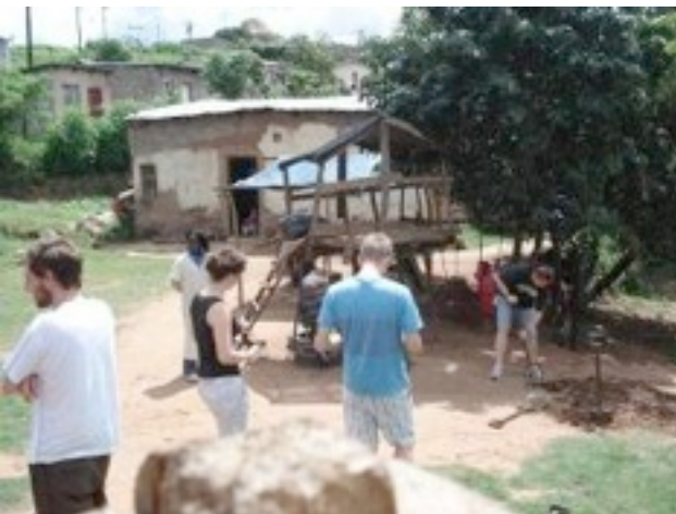
Laying grass at an underprivileged crèche in Mariannhill.
